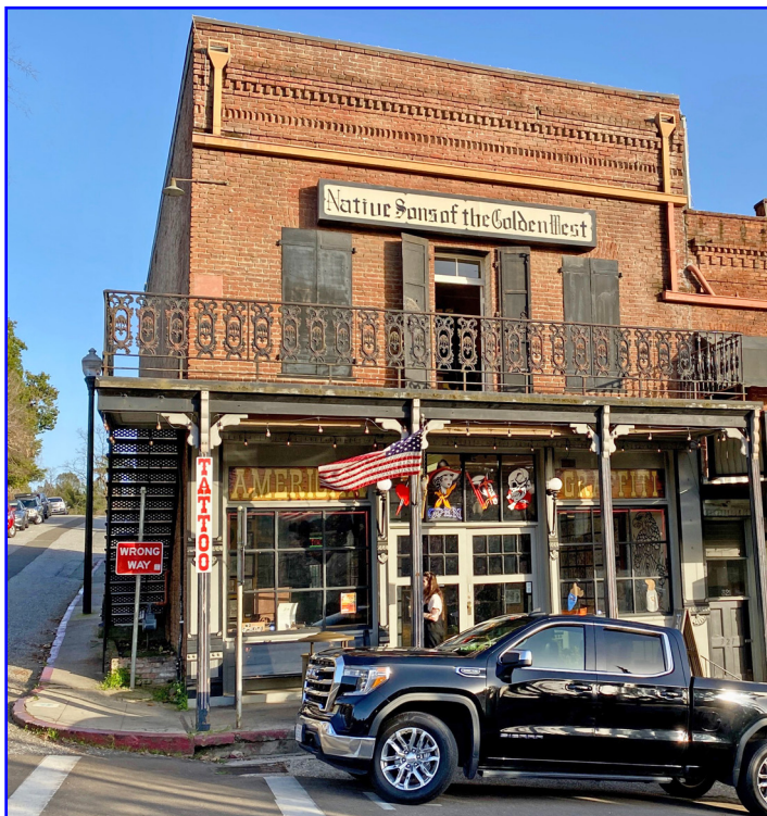
Auburn Parlor's historic hall.
